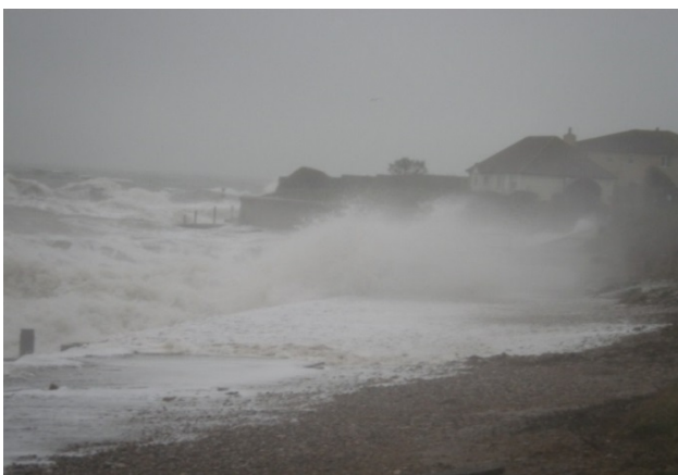
3. Overtopping at Selsey East Beach 14 th December 2012
