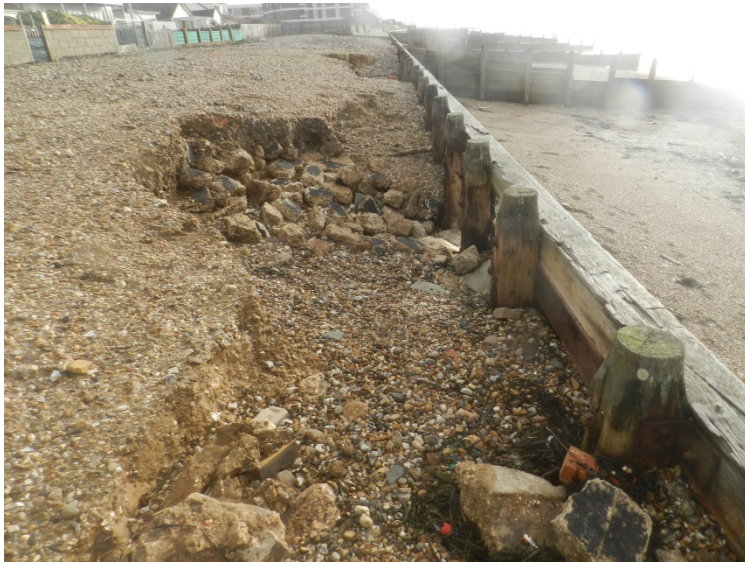
Photo 2.4: January 2014, Low beach levels at East Wittering causing undermining of timber breastworks.
